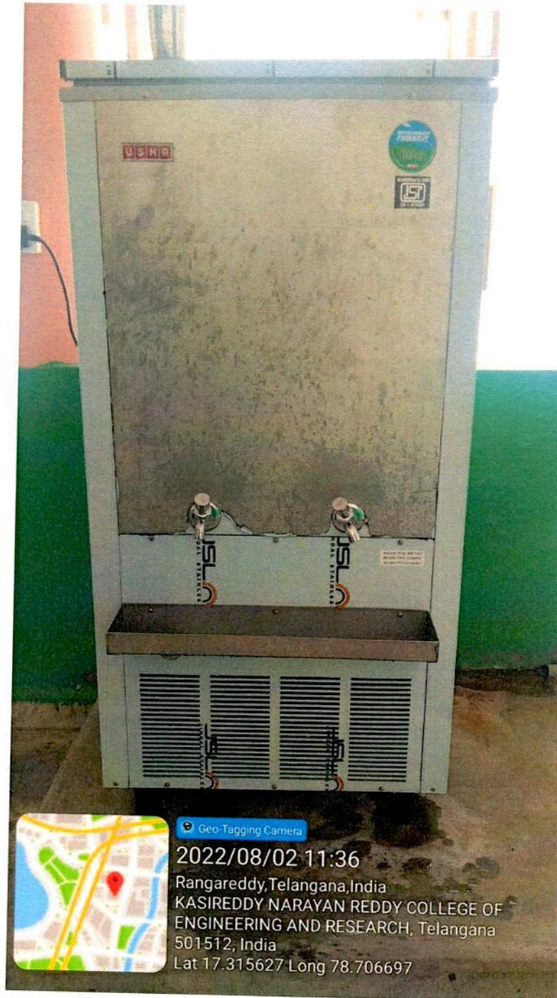
Final Water Distribution to Water-Freezers at KNRCER
